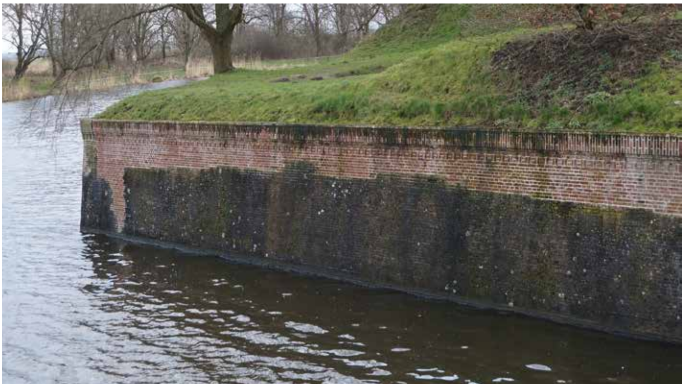
7.15) The masonry of the adjacent bastion (Katten), that was restored in 2009, still stands out very much in comparison to the older masonry. Besides that, this older masonry shows much more growth of moss and algae.
