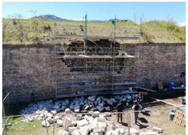
9.11) The crowning was reconstructed.
