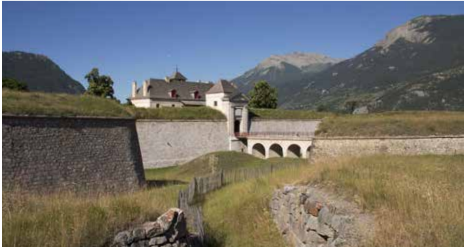
9.6) The Briançon gate.
