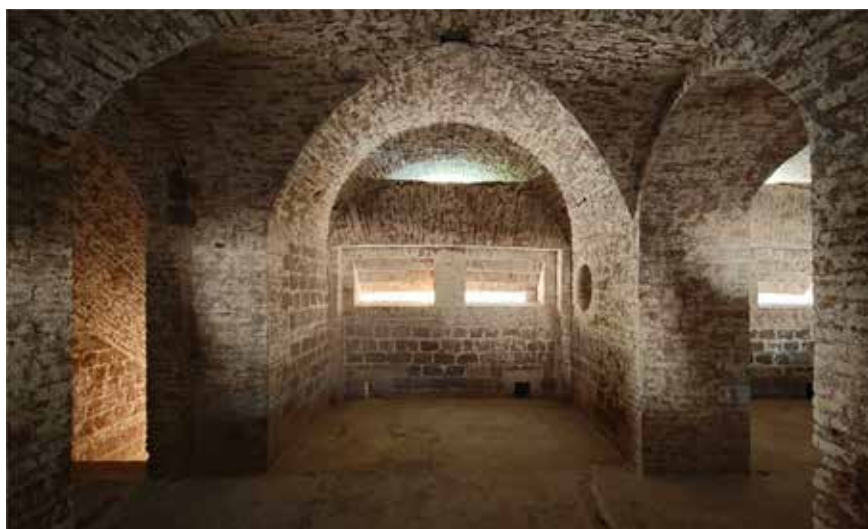
10.7) Interior of the central caponier.
