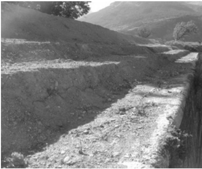
9.8) Embankment of the Briançon gate.
