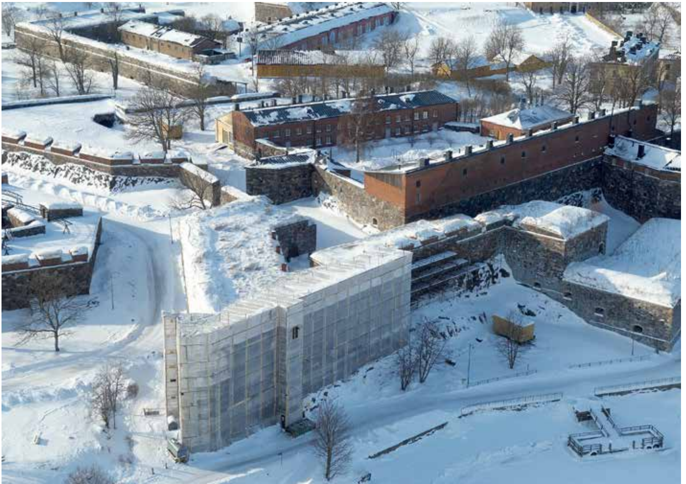
4.27) B48 Bastion Virtue (Hyve) under restoration 2010.
