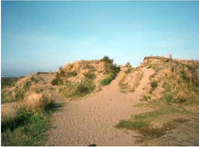
5.4) Picture has been taken in the 1970's when the ramparts were badly eroded. In some places we are going towards the same situation when the green surface of the ramparts is vanishing and the structure of sea sand layer is revealed.
