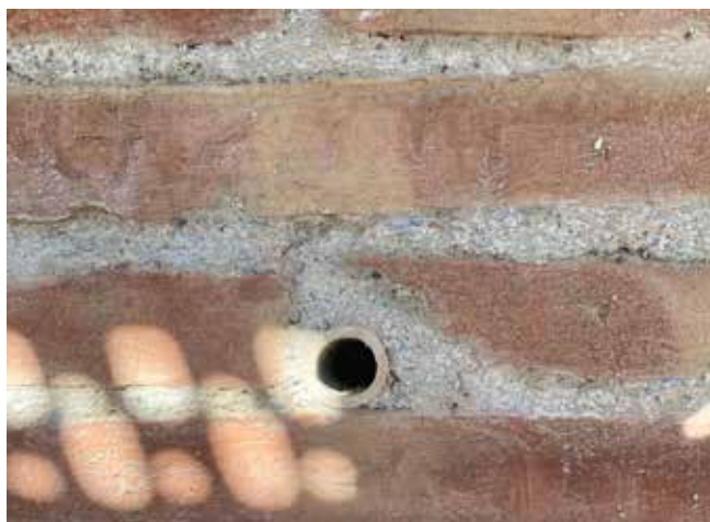
11.9) The restored brickwork in Antibes' rampart.
