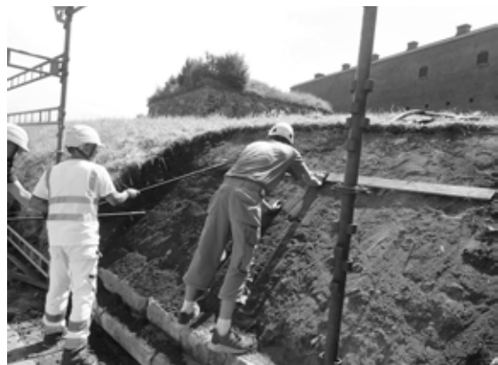
4.13-14) Rebuilding partly collapsing parapets in Bastion Wrede summer 2020.
