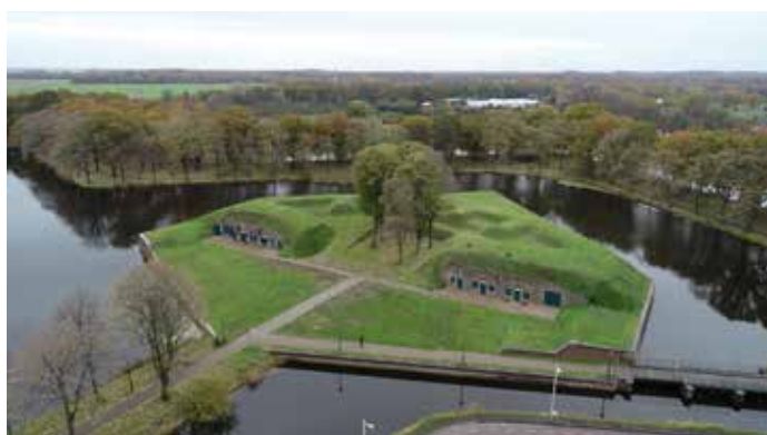
7.7) Aerial view of one of the ravelins in Naarden. The masonry of the ravelin dates from the 17th century. The earthworks of the ravelin were completely remodelled in the 19th century. At that same time (1875) the two bombproof guardhouses were constructed. They consist of a thick masonry construction, covered in an even thicker layer of earth.
