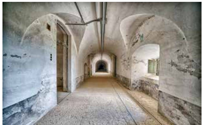
10.5) Interior view at the level of the armoured batteries.
