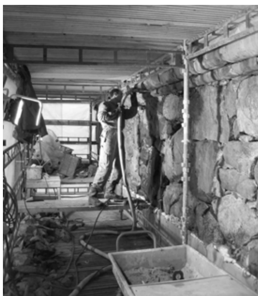
4.16) Grouting is a common method used in Suomenlinna wall repair.
