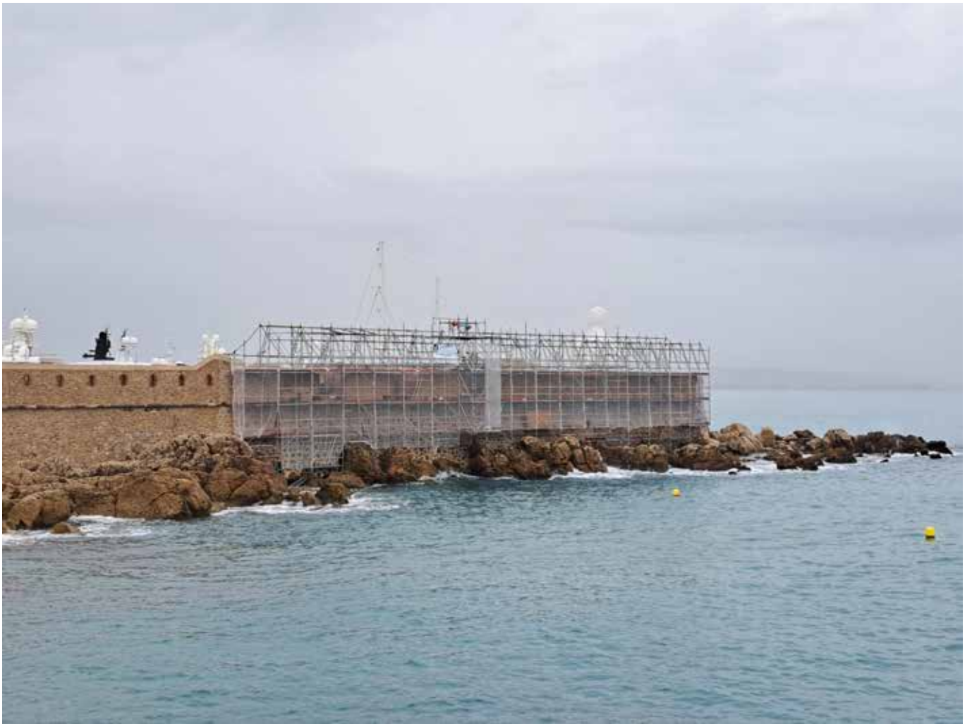
11.4) Scaffoldings for the first phase of works.
