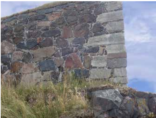
4.28-29) The two faces of the salient of A5 bastion Gyllenborg were restored in 2005 and 2006 with hydraulic lime mortar. In the photos taken in 2021 it is clearly visible that the left face of the bastion already needs repair. It is orientated to southwest (open sea) receiving wind, rain and sun. The increasing number of freeze-thaw cycles shortens the restoration life cycle of Suomenlinna fortifications.
