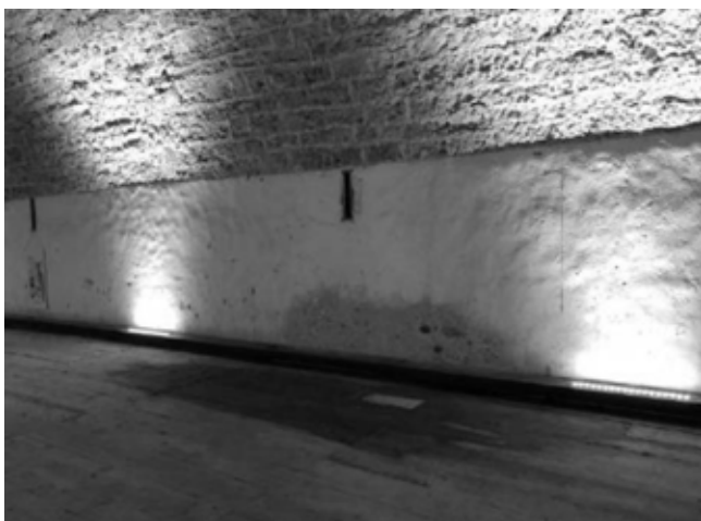
9.12-13) Infiltrations in the powder magazine.
