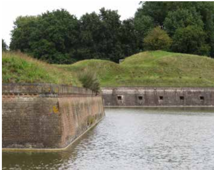
7.5) Picture of the 17th century fortifications, showing the embrasures of the five casemates in one of bastions. From here the ditch around the ravelins (on the foreground) could be defended.
