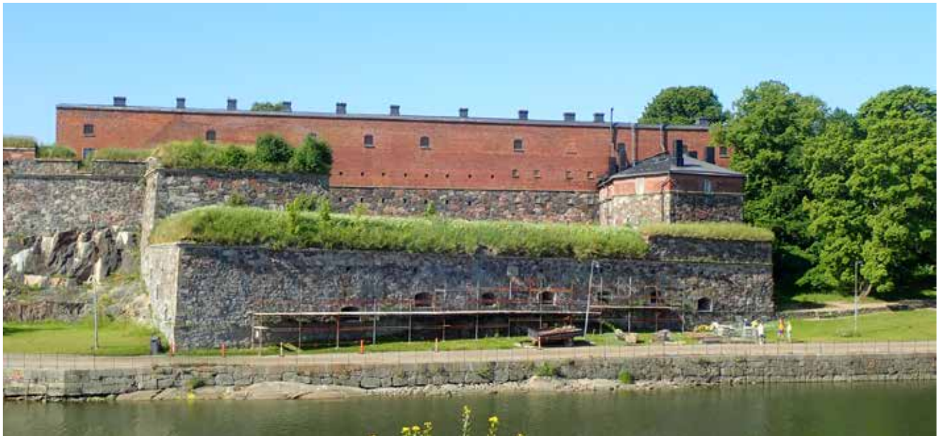
4.11) Construction site of Bastion Wrede in summer 2020.
