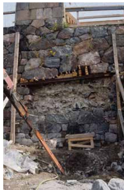
4.2-3) In 1980s the restoration methods were often maximum interventions. In 1990s, in the case of A13 shore work, only the parts in bad structural condition were repaired.
