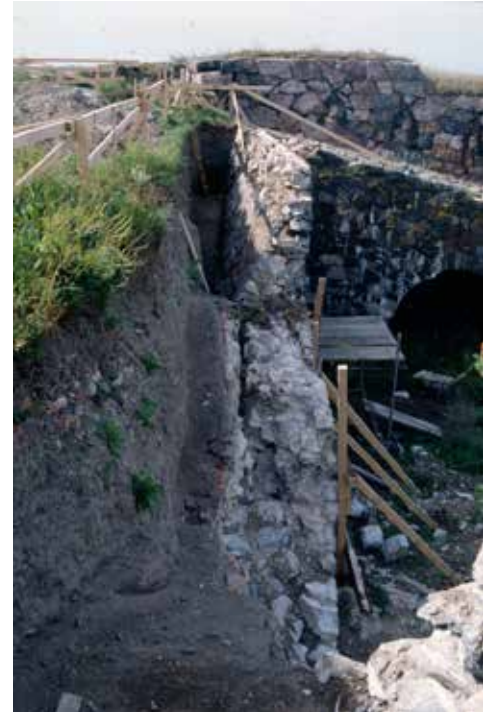
4.18-19) Earlier all earth was removed before restoration work. In A13 shore work restoration project only the soil hindering repair works was removed.
