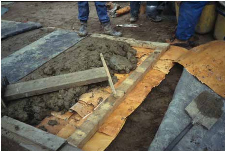
4.8) Coming from a Pelso prison in the Oulu region, the birch bark was harvested from trees that were going to be cut at the end of June or beginning of July. The clay was found near Helsinki from an old brick factory's land.
