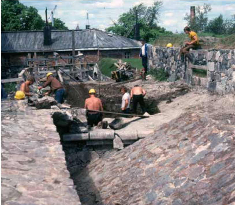
4.18-19) Earlier all earth was removed before restoration work. In A13 shore work restoration project only the soil hindering repair works was removed.
