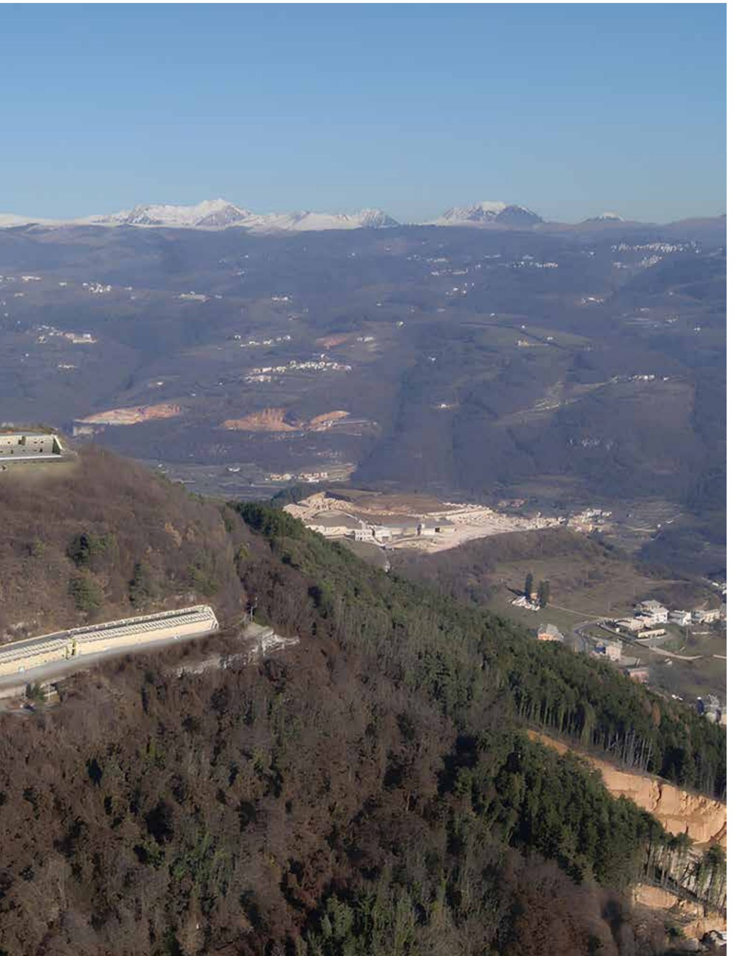
10.1) Aerial view of the Forte Tesoro and barracks after the restoration project.
