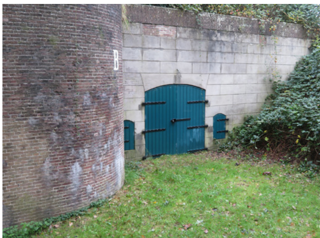
Figure 3. Naarden (NL), the building made of lime-based concrete dating from 1878 (Authors).
