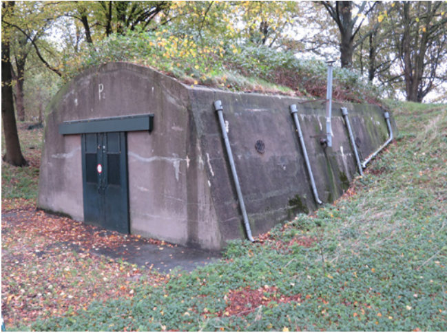
Figure 6. Naarden (NL), concrete shelter on the covered way dating from 1895. The drainpipes were added in a later restoration (Authors).
